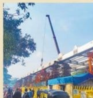
The girders of the Vidyavihar road overbridge are almost complete
