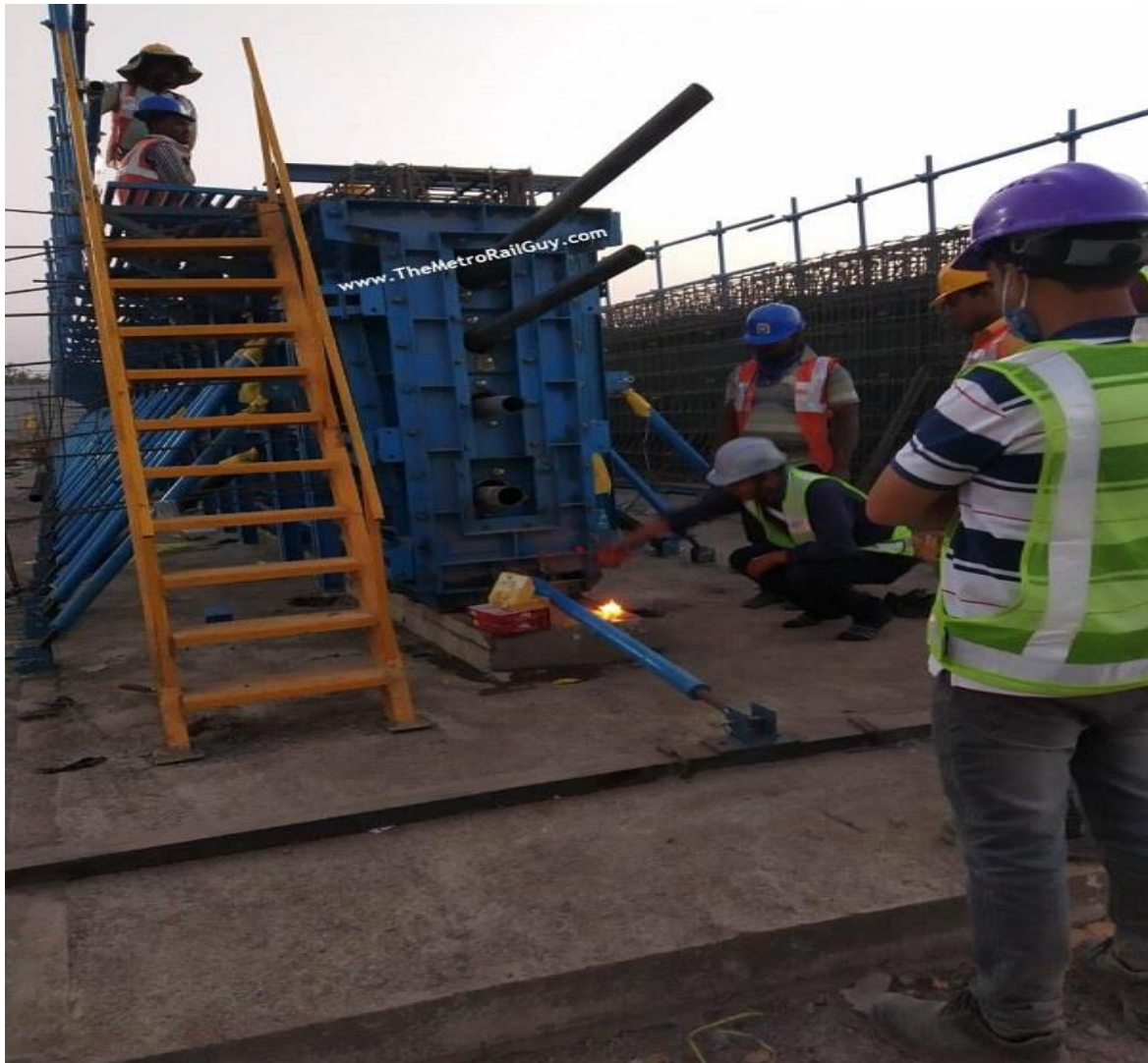
puja prior to pouring concrete
